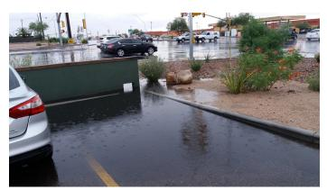
Fig. 18. Insufficient drainage into the basin.
