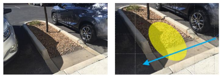
Fig. 24. With this design, water flows (blue arrow) past the planter due to the elevation of the concrete slab and the soil. For effective water infiltration, the concrete slab and soil (yellow oval) should be lower than the curb inlet and outlet.
