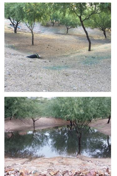
Fig. 16. Large detention basin without (above) and with runoff (below) after a rain event.
