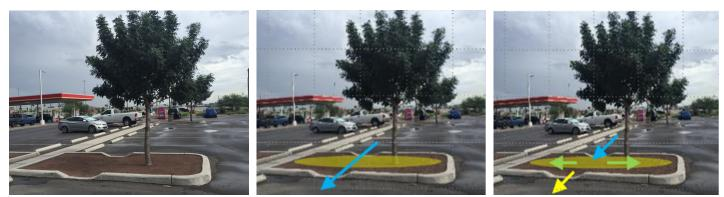
Fig. 25. Water harvesting in this planter is not effective and can be optimized by lowering the soil surface level.
