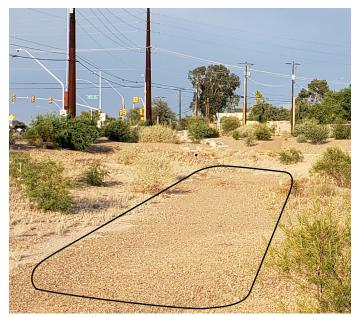
Fig. 11. Infiltration basin (inside black line) with scarce access by plant roots.
