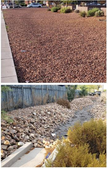
Fig. 9. Runoff from the parking lot flows into a large, shallow basin (above) and into a smaller basin (below).
