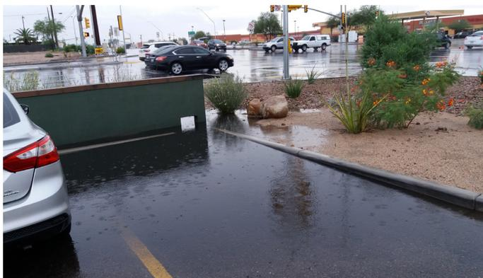
Fig. 18. Insufficient drainage into the basin.
