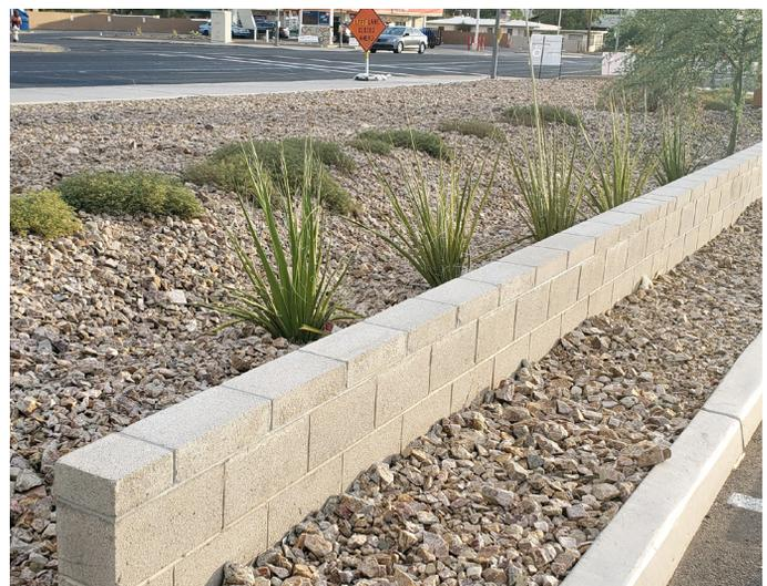
Fig. 23. Narrow infiltration basins
