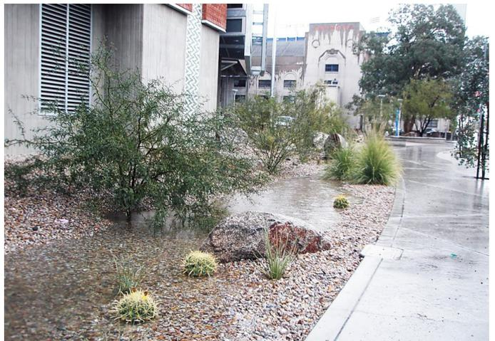
Fig. 4. Plant placement adjacent to infiltration basins
