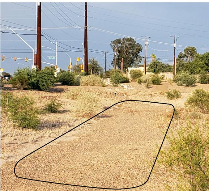
Fig. 11. Infiltration basin (inside black line) with scarce access by plant roots.
