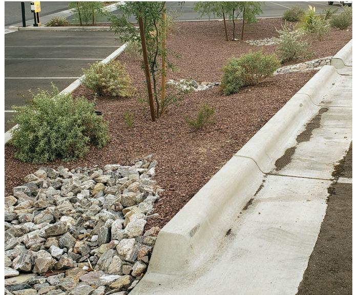
Fig. 8. The design and installation of this infiltration basin captures runoff from the parking surface through several curb inlets which are secured with rocks to prevent soil erosion.
