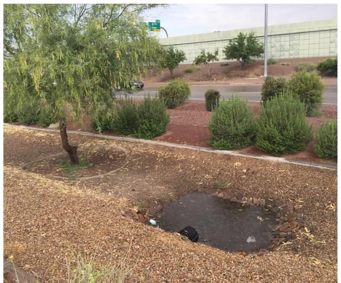
Fig. 21. Parallel placement of the infiltration basin to the tree supplements the root zone of the tree without excessive moisture at the trunk base.
