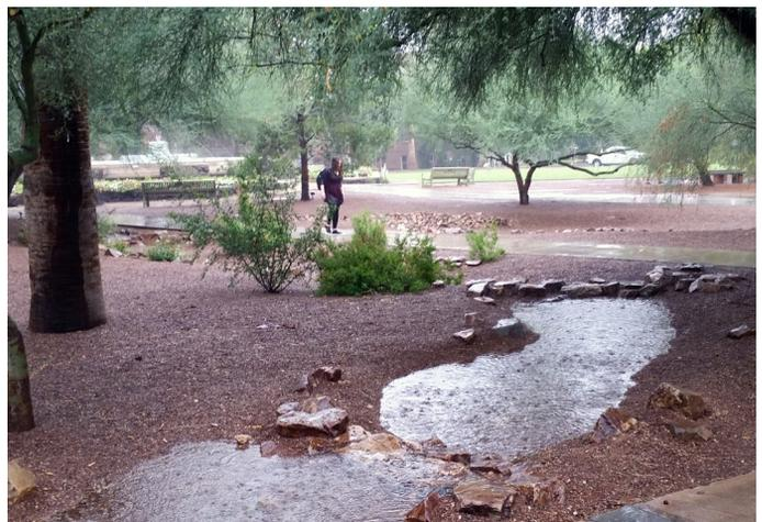
Fig. 5. Check dams separate infiltration basins.
