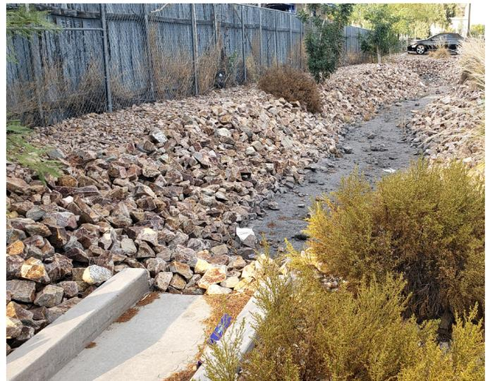
Fig. 9. Runoff from the parking lot flows into a large, shallow basin (above) and into a smaller basin (below).
