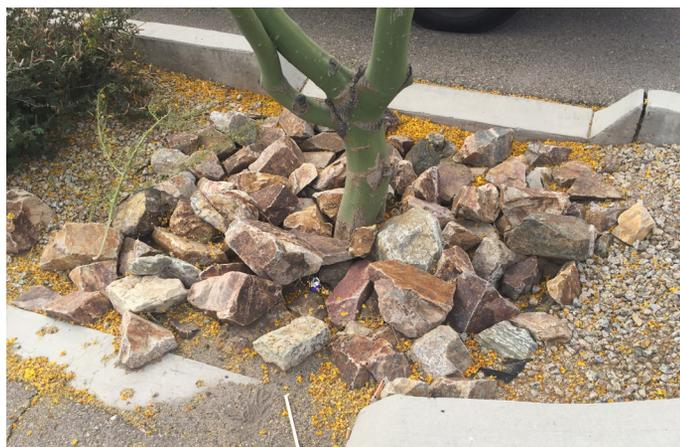
Fig. 15. Parallell curb cuts in a small planting island and riprap on top of the tree root zone.
