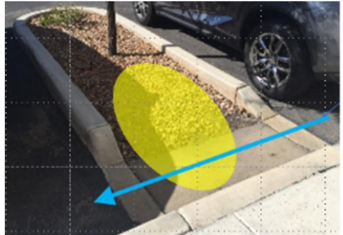
Fig. 24. With this design, water flows (blue arrow) past the planter due to the elevation of the concrete slab and the soil. For effective water infiltration, the concrete slab and soil (yellow oval) should be lower than the curb inlet and outlet.
