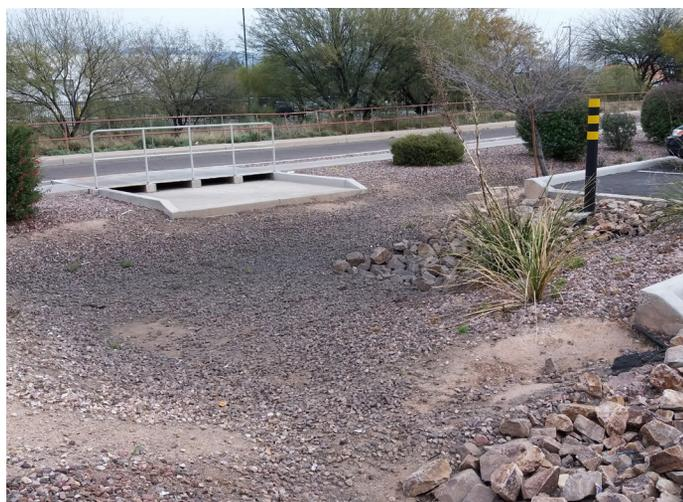
Fig. 19. This large, deep basin will overflow into a culvert to prevent flooding of the adjacent street.
