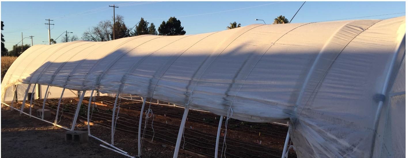
Fig. 5. Hoop house sides are raised in the morning for ventilation and closed at the end of the day.
