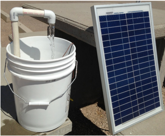
Figure 2. A solar module powers a DC bilge pump to move water. An example of a simple, or PV direct system.
