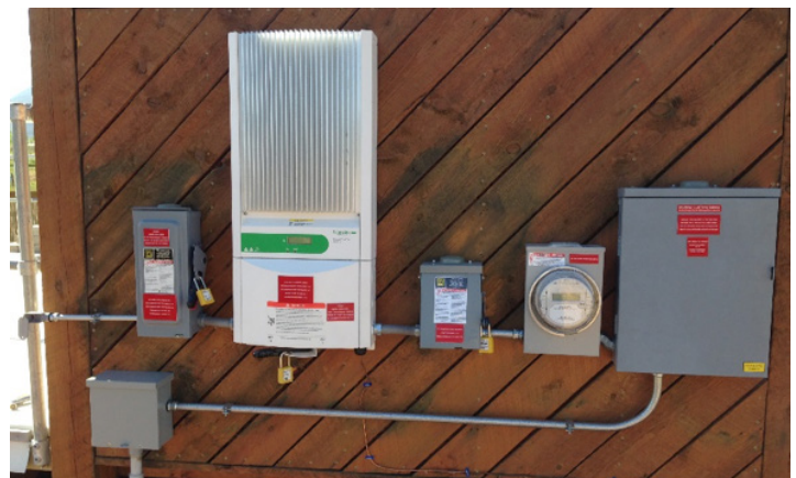
Figure 11. Example of a "balance of system" (BOS) of a grid-connected system. Components include safety disconnect switch on the DC-side, the inverter, a safety disconnect switch on the AC-side of the system, a meter, and the service distribution panel.
