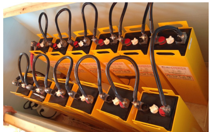
Figure 9. A bank of batteries connected together in series (wired positive to negative) to build voltage. The batteries are housed in a vented enclosure.
