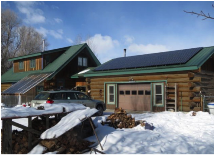
Figure 3. In a higher elevation, the array needs to be mounted so snow is not piling up on the edges of the modules. Courtesy Nunatak Alternative Energy Solutions
