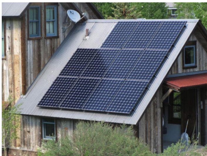
Figure 1. A roof mount array on a pitched roof. There is open roof space on all sides of the array for access. The empty space is next to the roof vent. Courtesy Nunatak Alternative Energy Solutions
