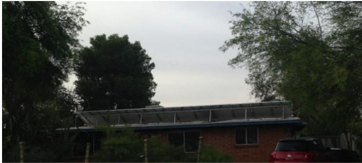
Figure 4. Tilt-up mounting systems on low slope or flat roofs are a method to set the tilt of the array to the latitude of the location to maximize the energy output of the array. Although this system is facing south, shading cast on modules from nearby trees can limit the amount of energy an array is capable of producing.
