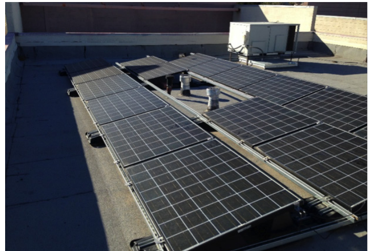
Figure 9. An array mounted on a flat roof of a commercial facility. Shade from a nearby wall is cast upon a portion of the array.
