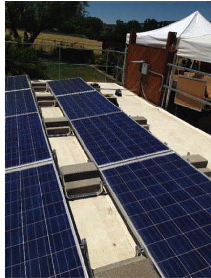
Figure 8. Ballast mounting systems rest on the surface of the roof and are held in place with cinder blocks. Modules are clamped to the aluminum frame at an angle of 10 degrees.
