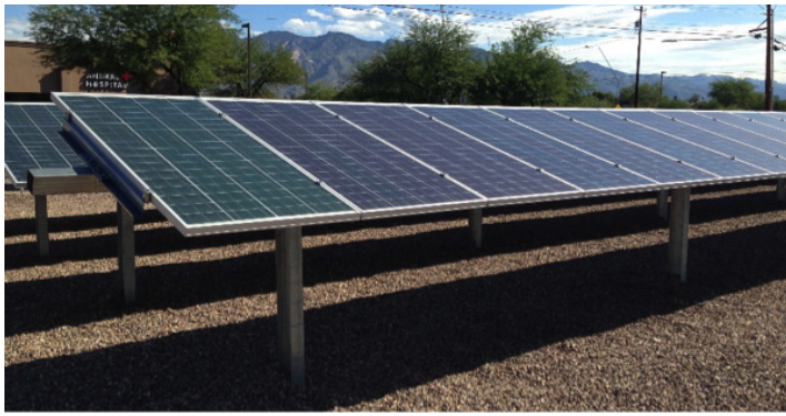
Figure 6. A ground-mount system requires space for installation. The size of the modules and array will impact the size and type of mounting system materials. Accessibility for maintenance, and air circulation for cooling modules are an advantage of this type of mounting system
