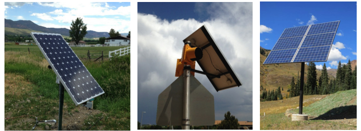
Figure 5. Modules or array affixed to a rack and mounted on the top of or to the side of a pole. The pole-mount can be oriented in a specific direction. The amount of excavation depends on the size of the array.
