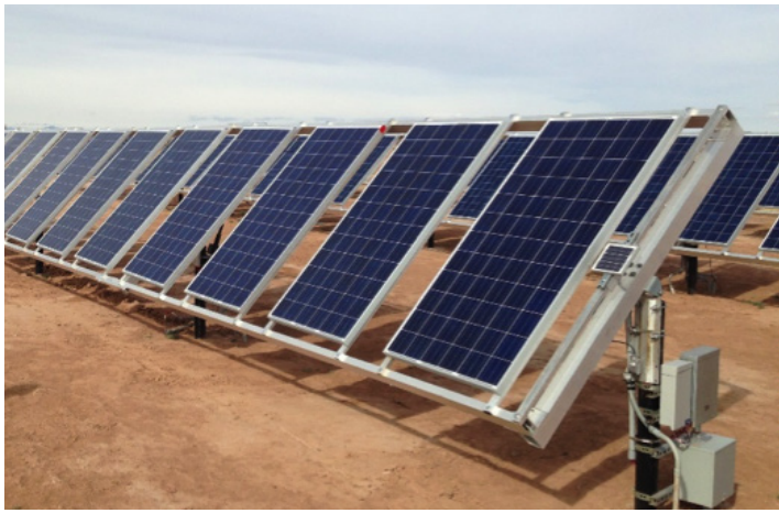
Figure 10. A ground-mount system with a north-south tracking capability to keep the array perpendicular to the sun. Array tilt can be set to latitude during spring and fall, and adjusted 15 degrees during the summer (latitude – 15 degrees) and the winter (latitude + 15 degrees).
