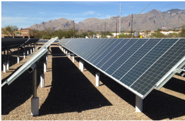
Figure 11. An east-west tracking commercial-sized array. A hydraulic ram pulls and pushes a rod connecting multiple rows of arrays. The array position begins facing the east in the early morning. The array moves a slight bit every 15 minutes to follow the sun as it crosses the sky. At sun down, the array is repositioned to face the east.
