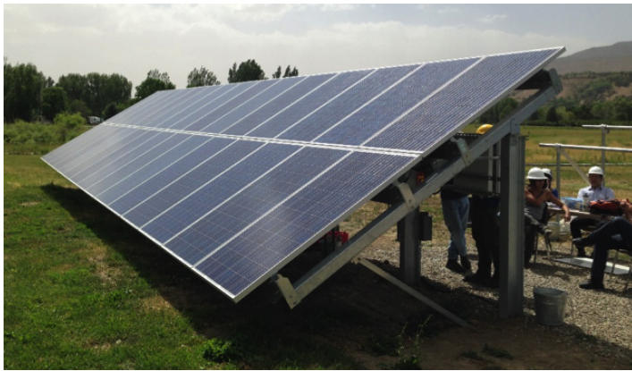
Figure 7. Solar modules arranged in two rows on a large fixed-plate ground mount system. The larger size modules require larger mounting materials to support the weight and to keep the system stable during high wind winds and at a tilt angle to allow snow loads to be easily removed.
