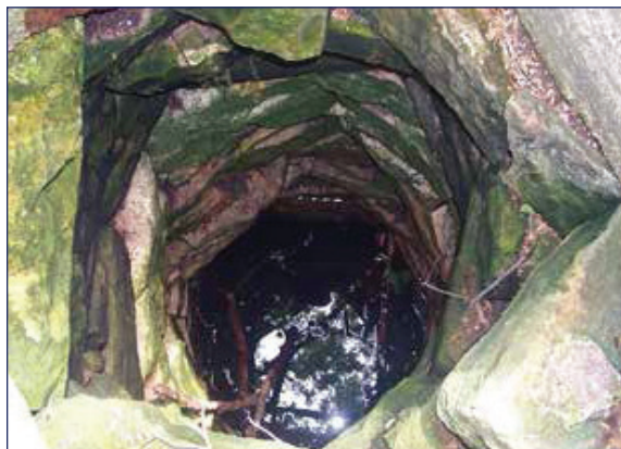
FIGURE 10.4 Unplugged, abandoned wells can be a source of groundwater pollution and maybe a safety concern.
