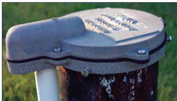
FIGURE 5.4 Example of a well cap made of aluminum.
