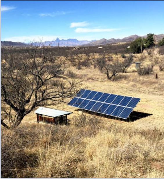
Domestic well powered by Solar cells.
