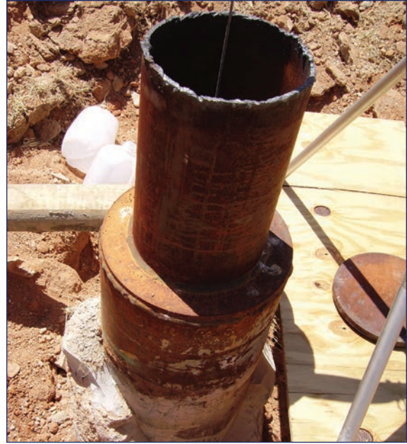
FIGURE 5.3 Photo of the sanitary seal grout around the surface casing of a well in construction.
