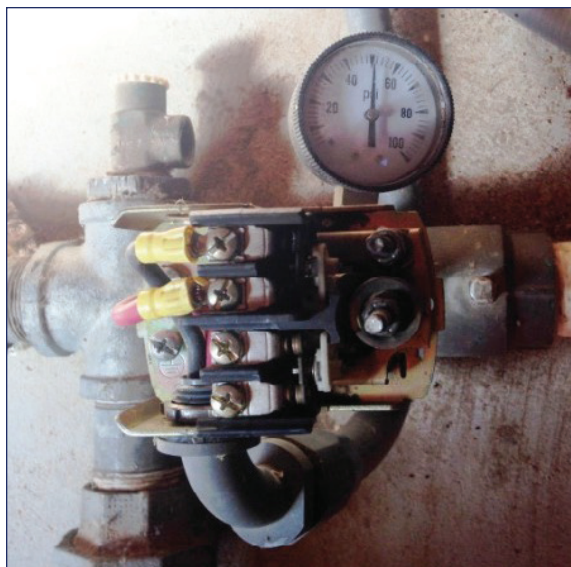
FIGURE 5.8 Captive air bladder tank pressure switch.
