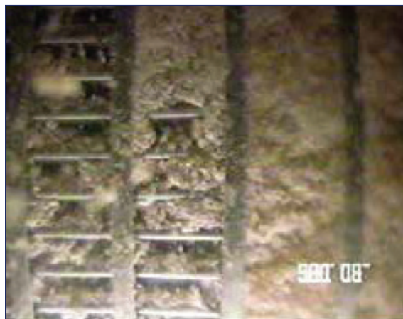
FIGURE 6.2 Scale formation on a well screen.
