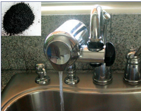
FIGURE 9.7 An activated carbon point-of-use treatment installed on a faucet; the carbon media is shown in the photo insert.
