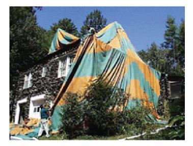
Then a fumigant gas is released into the structure. The gas penetrates into cracks, crevices, void areas and directly into wood to kill termite colonies. Lethal concentrations are contained by the tarpaulins long enough to permit uniform penetration deep into all infested areas.
