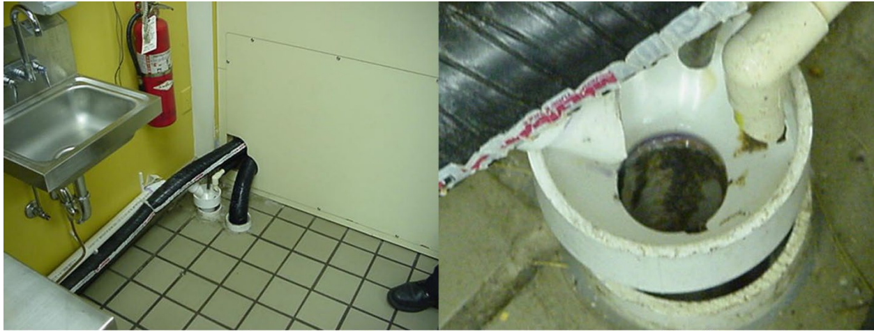
Figure 13. Condensate lines generate biofilms which support some fly species.
