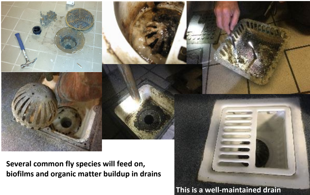
Figure 14. Five of the drains above were poorly maintained and generating fruit or moth flies. The drain on the lower right side is clean and was not serving as a fly resource.
