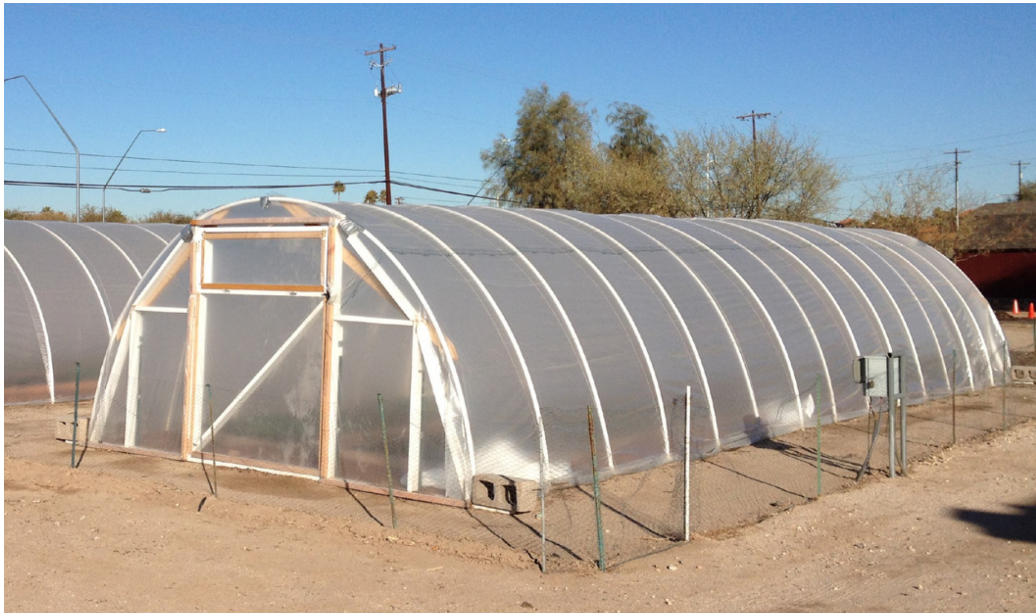
High tunnel with end-walls (photo by University of Arizona).
