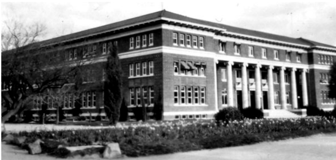
University of Arizona, Forbes Building (built in 1915) which is home to the College of Agriculture and Life Sciences in Tucson.
