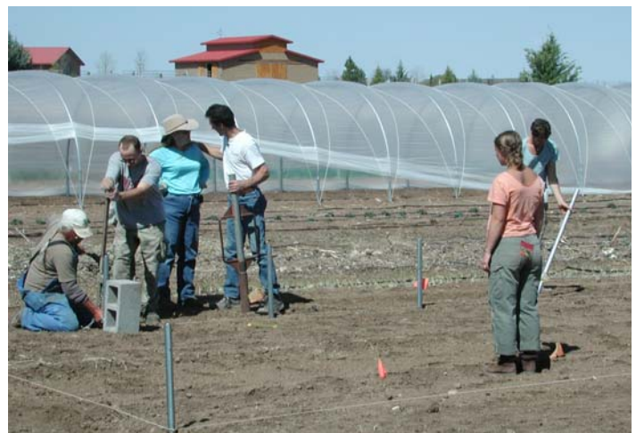
Beginning Farmers laying out a hoop house prior to construction. A completed hoop house is visible in the background.
