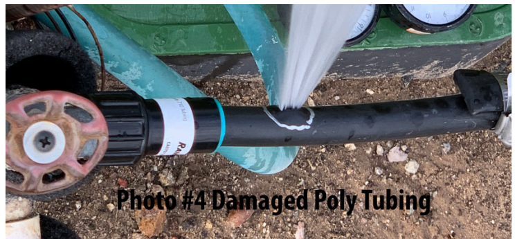
Example 3: Coyote puncture damage to 1/2 inch poly tubing. It is amazing how much water can pass thru a little puncture split in the tubing. Actually tested at 4.9 GPM. The photo shows the damaged section of tubing under test conditions (Photo 4).
