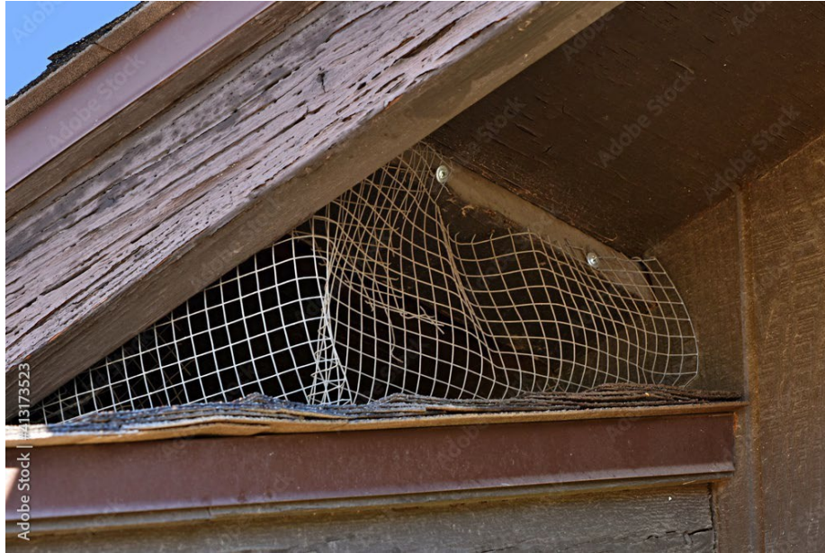
Figure 9. Pest-proofing is the best way to keep rodents out. Photo: Adobe Stock Images.
