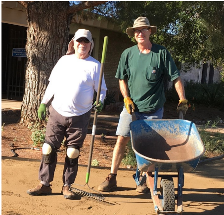
Master Gardener Volunteer Bill Guina(left) & Jeff Oesterle(right) from Oest Metalworks install the new path.
