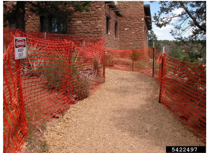
Temporary fence and heavy mulch preclude damage and mitigate soil compaction (Jason Sharman, Vitalitree, Bugwood.org).
