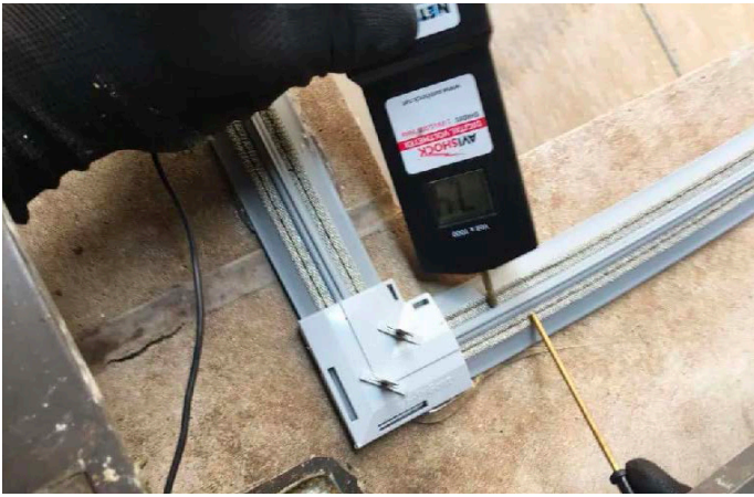
Figure 21. Electric shock track placed along ledges of buildings will prevent birds from landing. Photo: Standard Pest Management, Astoria, NY
