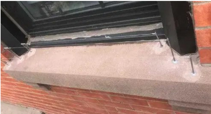
Figure 15. Well-placed bird wire is almost invisible and prevents pigeons from landing. Photo: Standard Pest Management, Astoria, NY
