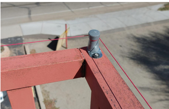
Figure 22. Electromagnetic pulse wire around a building perimeter. Photo: DaveFliesDrones.com
