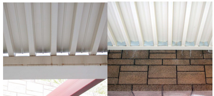
Figure 13. Roosting opportunity (left) and after pest-proofing measures are taken (right). Photos: Dawn H. Gouge, University of Arizona
