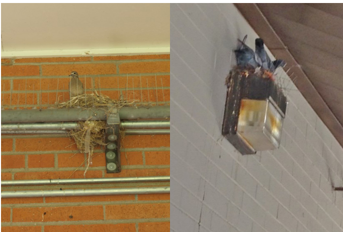
Figure 16. Not all perching places can be spiked successfully. Here a native dove is nesting behind bird spikes which have generated a nesting opportunity for a different bird species (left) and pigeons (right). Photos: Dawn H. Gouge, University of Arizona
