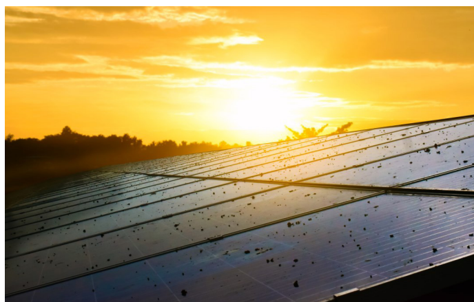
Figure 9. Pigeon droppings on solar panels, which reduces efficiency. Photo: Shutterstock
