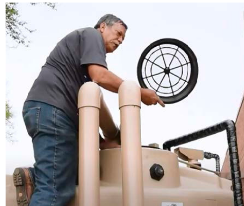
Figure 5. Basket strainer fits into a cistern manhole lid. Photo courtesy of Oasis Water Harvesting.
