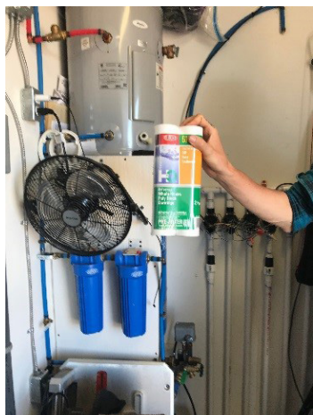
Figure 12. Sediment filters need to be changed every three months. Photo courtesy of Derek “Handeeman” Howlett.
