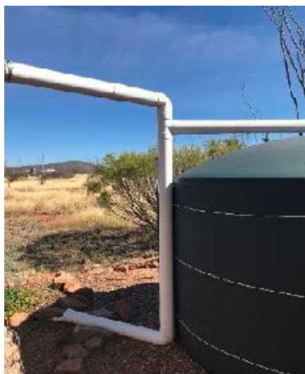
Figure 3. A first flush diverter. The angled pipe on the left brings water from the roof. The vertical pipe, along the left side of tank, diverts the first, dirtiest water. The horizontal pipe on the right is the inlet pipe taking cleaner water to the tank.
