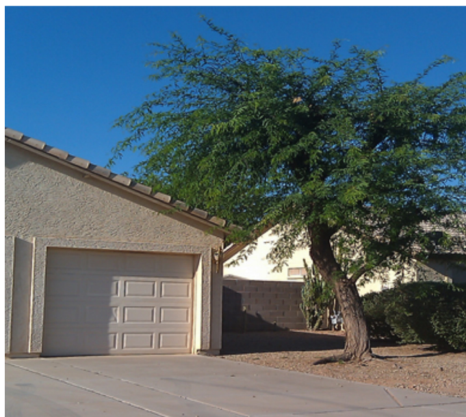
Figure 4. Tree branches rubbing on the tile roof of a home and lopping over into the yard of a neighbor caused the owner of the tree in the photograph to prune the tree heavily. Six months later, the tree is again creating problems.
