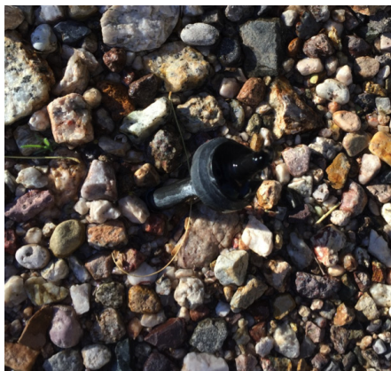
This drip emitter is connected to micro-tubing which is attached underground to a lateral line..
