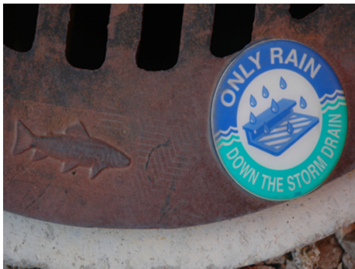
Figure 6. Storm Drain Marker in Tucson
