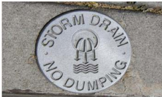
Figure 5. Storm Drain Marker in Maricopa County
