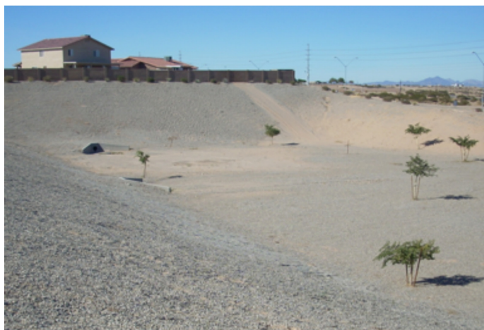
Figure 4. Stormwater Infiltration Basin in Yuma
