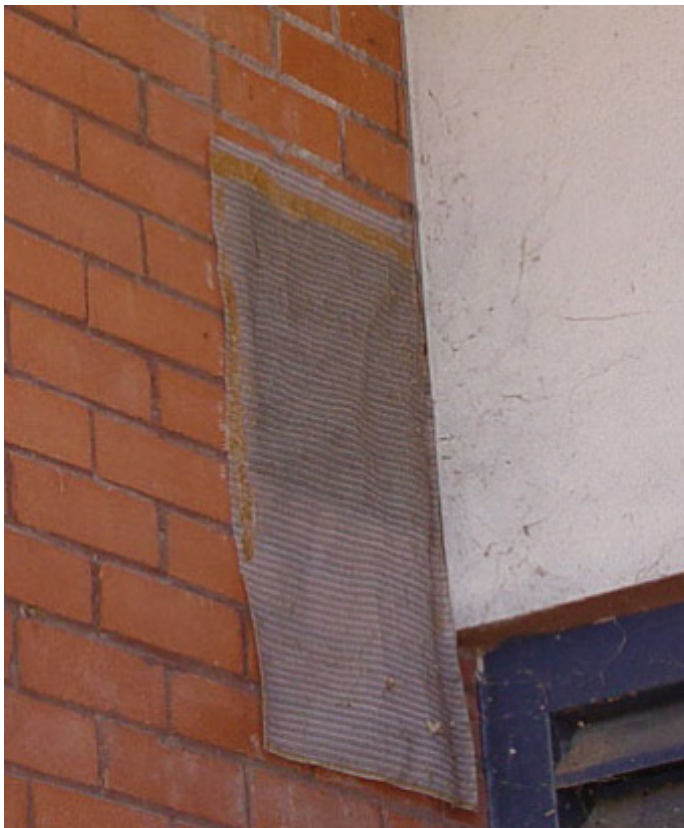
Figure 5. A one-way cover over holes allows bats to leave a structure but keeps them from getting back in. Photo by Nancy Renison.
