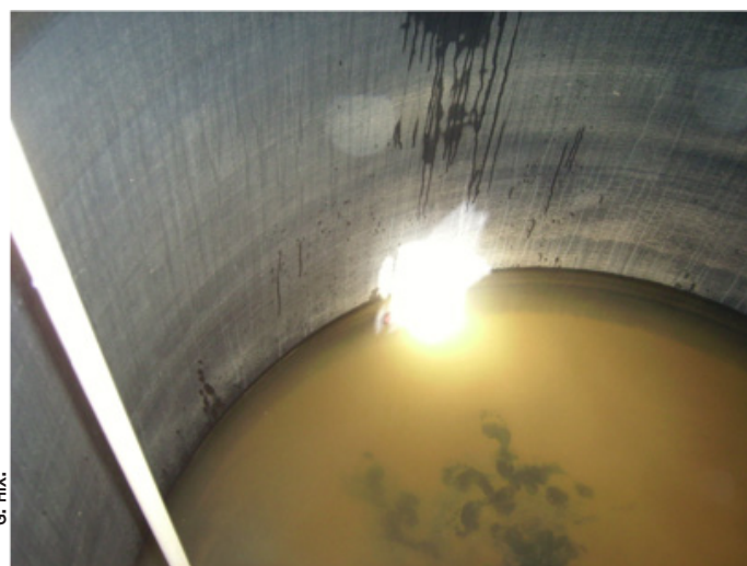
Figure 4. Inside a water storage tank nearly empty, sediment and algae growth visible.
