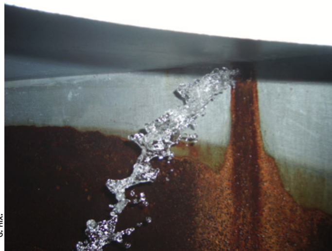
Figure 3. Inside of a water storage tank with visible rust.
