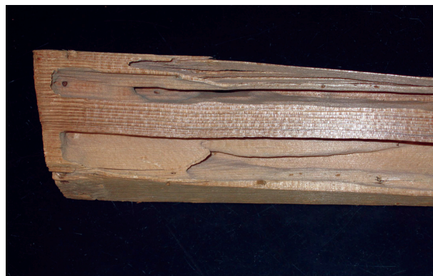
Fig. 9. Drywood termite damage.
