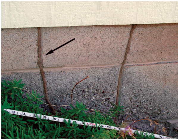
Fig. 12. Shelter tubes on a building foundation.
