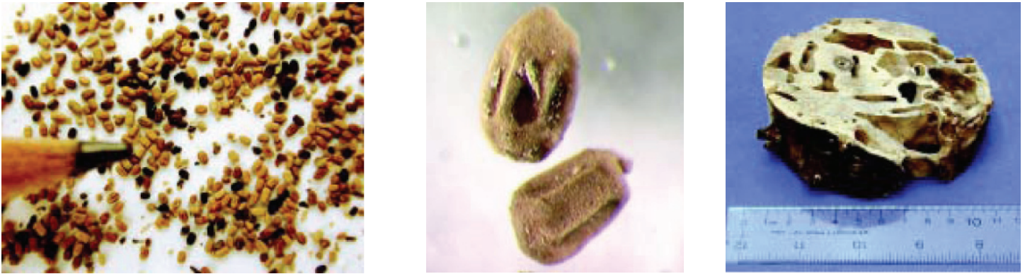
Figure 3. Drywood fecal pellets and damage
