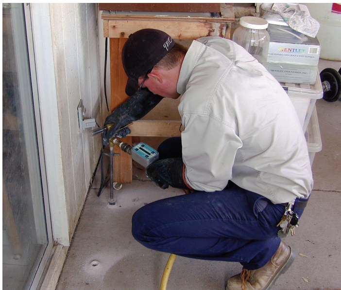
Figure 6. Application of termiticide into patio
