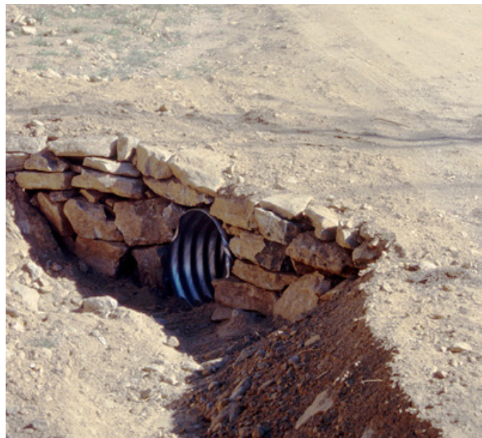
To be effective, culverts must be installed properly and at proper locations.
