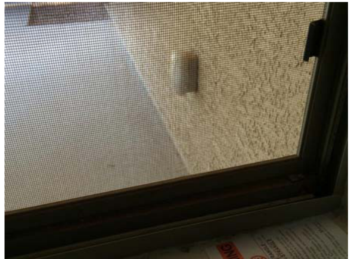
Fig. 5. Mesh screen installed on a window.
