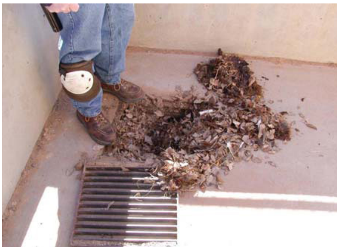
Fig. 14. Clean out grates and drain covers periodically.
