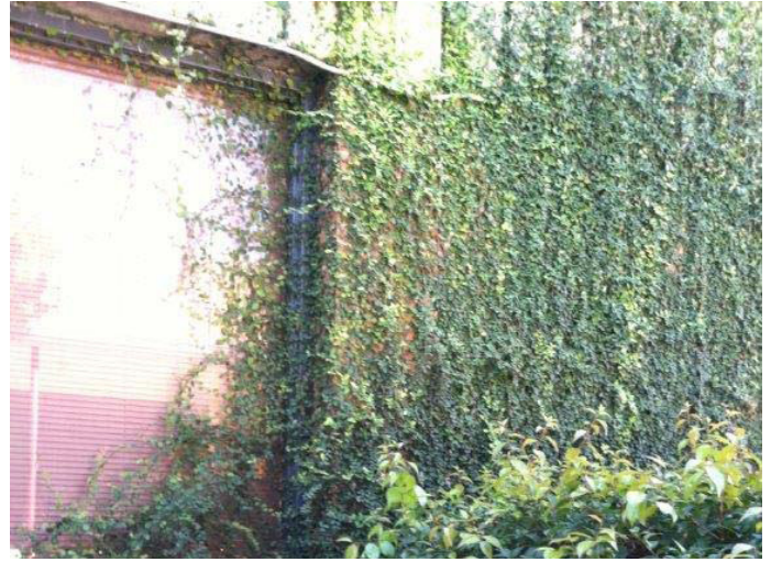
Fig. 15. Vines growing on the walls provide pests with access to the building.
