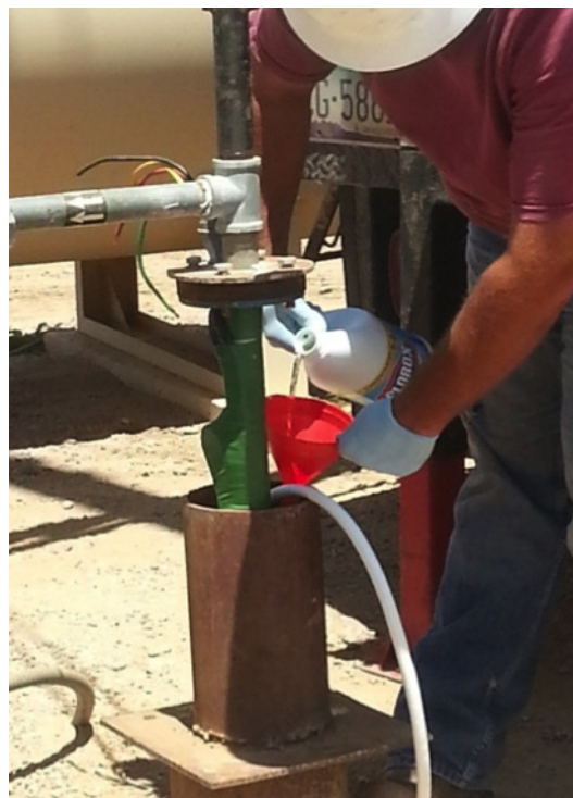
Figure 9. Contractor chlorinating a well. Note safety equipment and water circulation hose through the opened well seal, something most well owners cannot do themselves. Photo by G. Hix.
