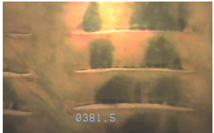
Figure 2. Louvered well screen covered with slime within days of being installed in new water well. Photo by G. Hix, 2012.
