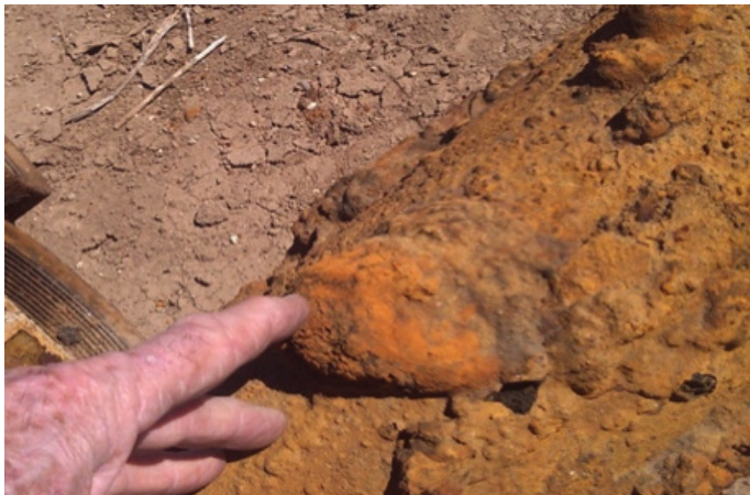
Figure 8. A water well pump encrusted with iron rust tubercles. Photo by G. Hix.
