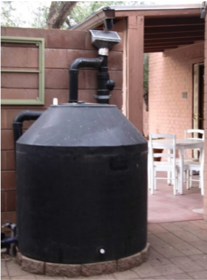
Figure 1. A cistern is placed under a gutter, where it collects rainwater from the roof. The screen and first flush device capture debris and pollutants.
